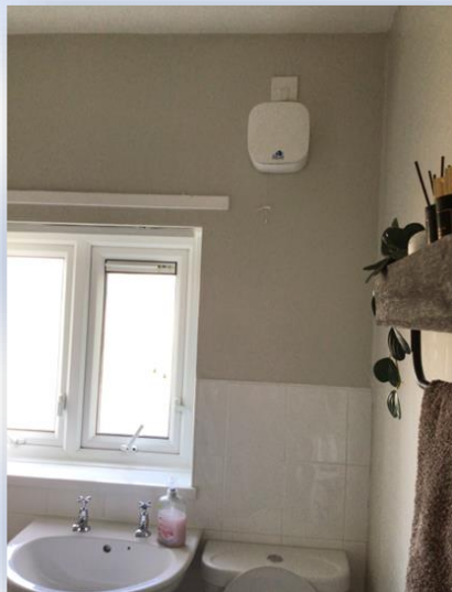
Replacement Bathroom Fan
